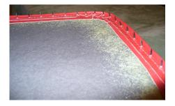
The back board is prepared for installation by pressing tacks through the bead edging
